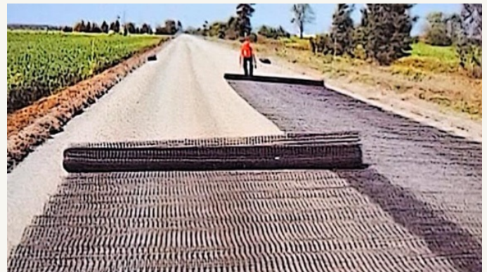
Roads & ground works
